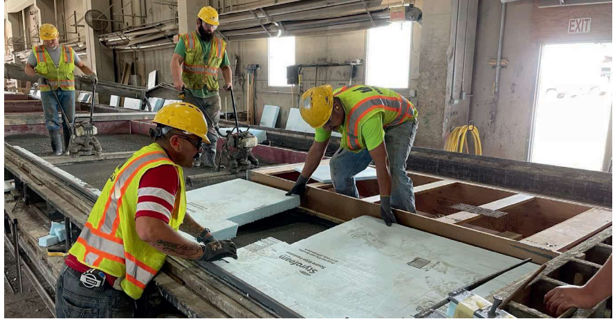
Workers at Wells Concrete manufacture support panels using wood forms.
