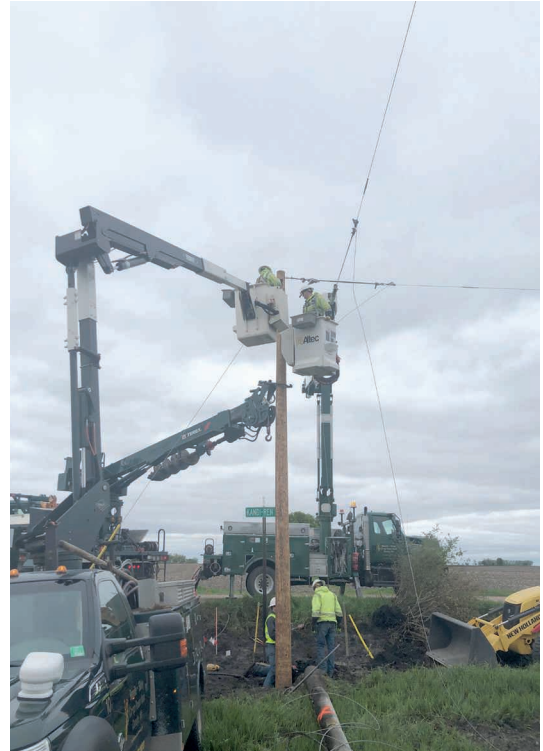
Renville-Sibley linemen replace a burnt pole.
